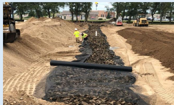
Figure 4.2: The TDA infiltration system at The Paynesville Secondary School during construction. (Park et al., 2023)
