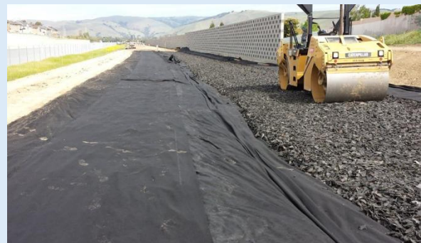
Figure 8.16: TDA was placed using a front-end loader and compacted with a smooth-drum roller.
