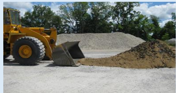
Figure 8.9: Loader bucket used to mix shredded tires and sand thoroughly.
