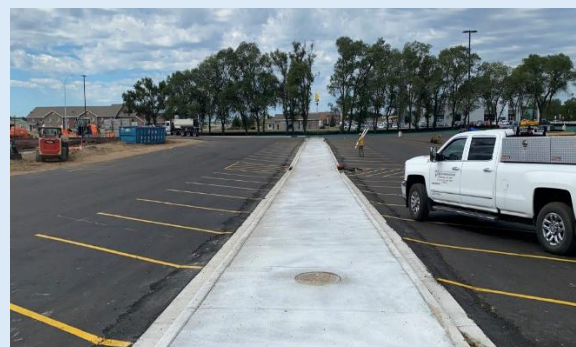
Figure 4.3: The TDA infiltration system at The Paynesville Secondary School after completion (Park et al., 2023).
