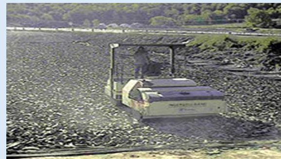
Figure 8.12: TDA spread in lifts of 12 inches.
