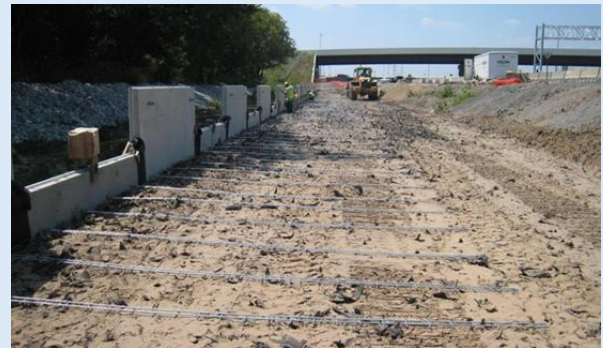
Figure 8.2: Mixture spreading in lifts of 12 inches using a bulldozer.
