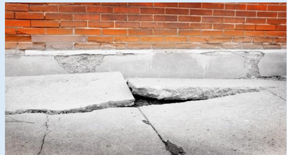
Figure 1.5. Damaged and uneven sidewalk due to frost heave.
