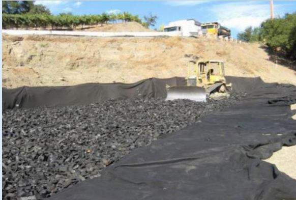
Figure 8.6: Placement of the TDA on the geotextile fabric during construction.
