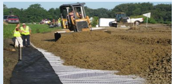
Figure 8.10: Mixture spread in lifts of 12 inches using a tracked bulldozer.
