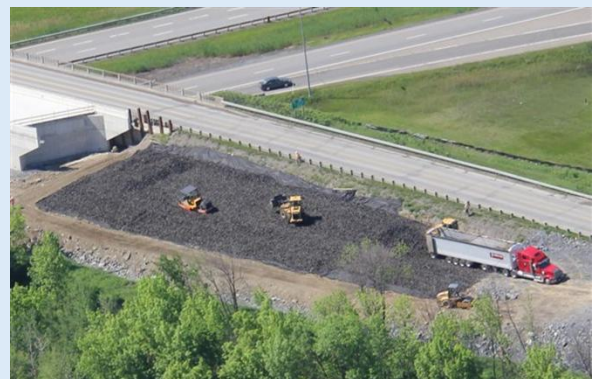
Figure 8.20: TDA was placed using a front-end loader and compacted with a smooth-drum roller (photo provided by Mr. Sangiuliano, MTO).
