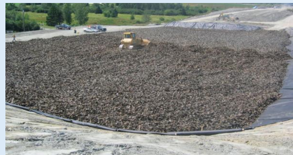
Figure 8.18: TDA was placed in 12-inch lifts using a front-end loader and compacted with a smooth-drum roller (after Mills et al., 2015).
