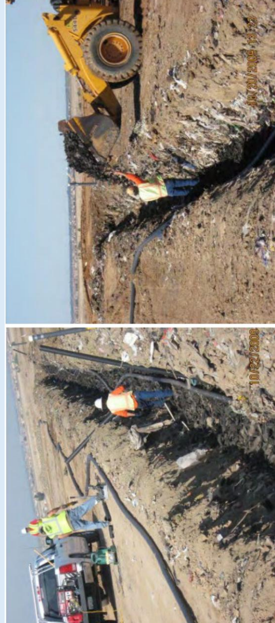
Figure 4.4: Installation of gas collection pipe and spreading TDA in the gas collection trench (Patenaude and Wright, 2011).
