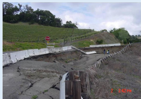
Figure 8.4: The landslide damage.
