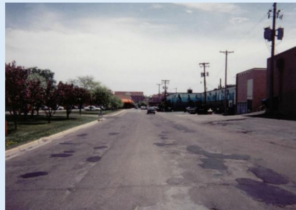
Figure 3.9: Extensive frost heave damage on Lake Drive in Robbinsdale, Minnesota. (TDA Manufacturing, 2024).
