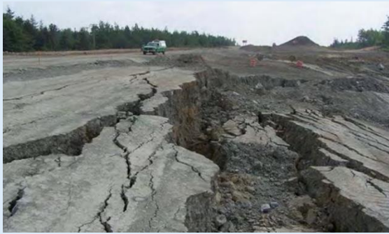
Figure 8.17: The St. Stephen embankment failure (after Mills et al., 2015).
