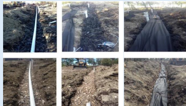
Figure 4.7: Trench installation stages
