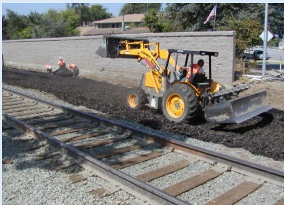
Figure 6.1: Spreading TDA during vibration damping installation for light rail (Cheng, 2016).
