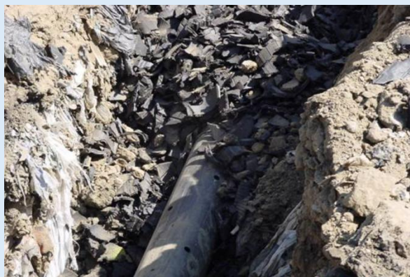
Figure 8.14: The gas collection pipeline covered in TDA material.
