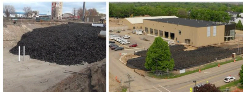
Stormwater Projects utilizing TDA
